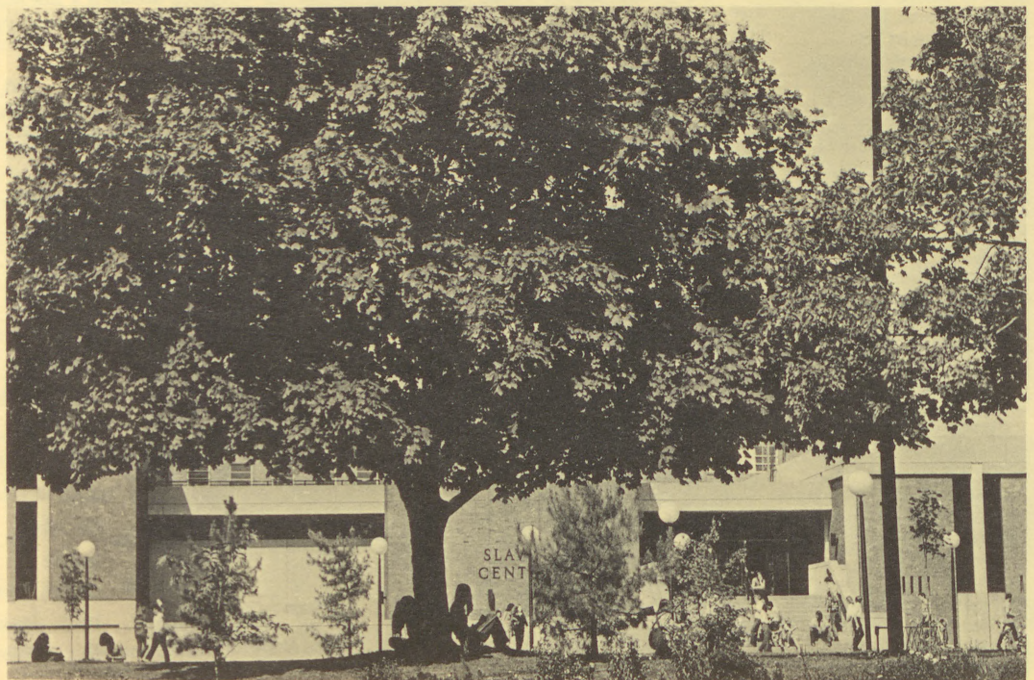
Slavin Center, a $3 million student union, was dedicated in 1973. The three level structure is named in honor of the late Very Rev. Robert J. Slavin, O.P., the college's sixth president.
