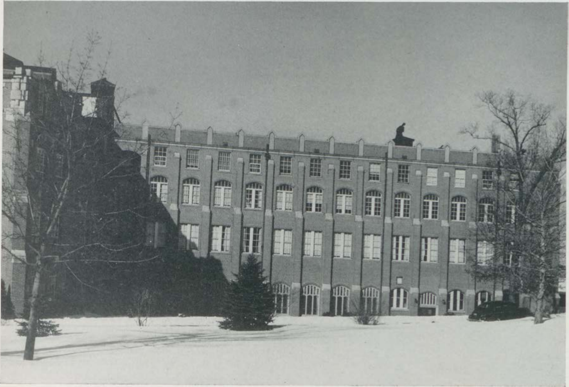
NEW WING TO HARKINS HALL was added in Fall of 1928, which practically doubled the original facilities. Auditorium and cafeteria on ground floor; second floor, class rooms and biology laboratories; third floor, library and chemistry laboratory; fourth floor, faculty living quarters.
